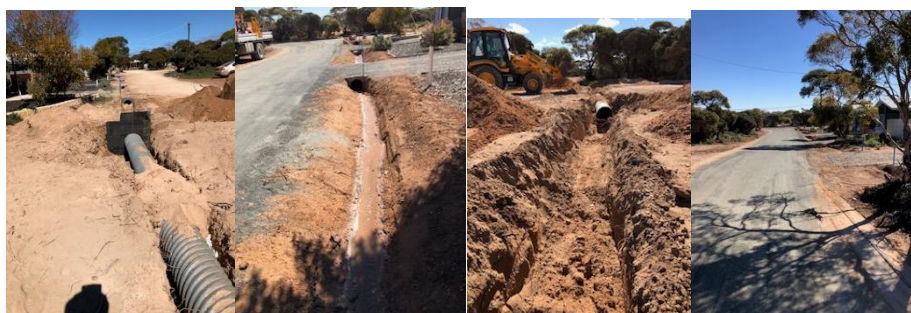
Culvert work carried out in Eucla.
