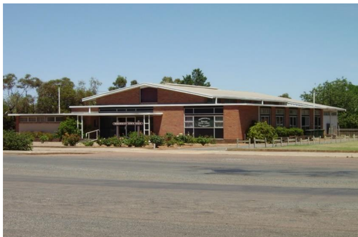
Shire of Dundas - TOWN HALL
